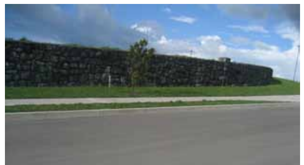
12. The stone retaining wall at Lynley Park is attractive and should be the preferred retaining option
