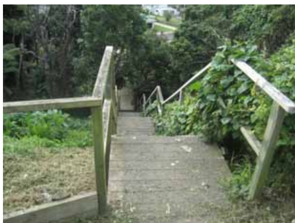
27 Remove the vegetation along the hand rail and erect a sign the warn the public not to use the walkway at night
