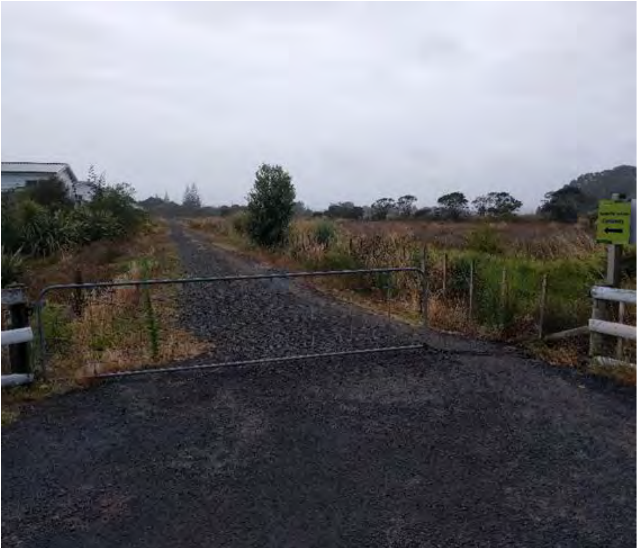
Figure 20 - View SE away from Emerton Rd along existing formed section
