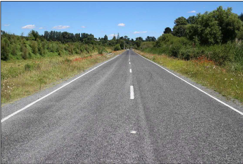
Photograph 3: Te Puna Station Road Looking West
