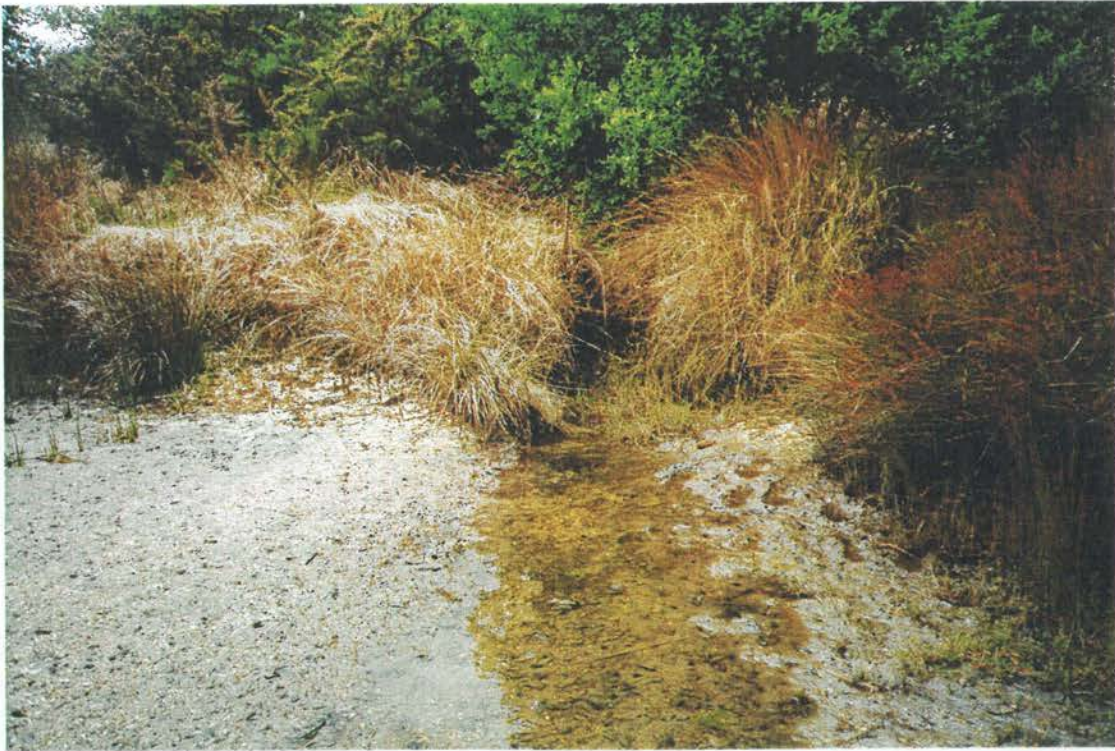
Plate 5: Site TN3 - Stormwater outlet at estuary margin.
