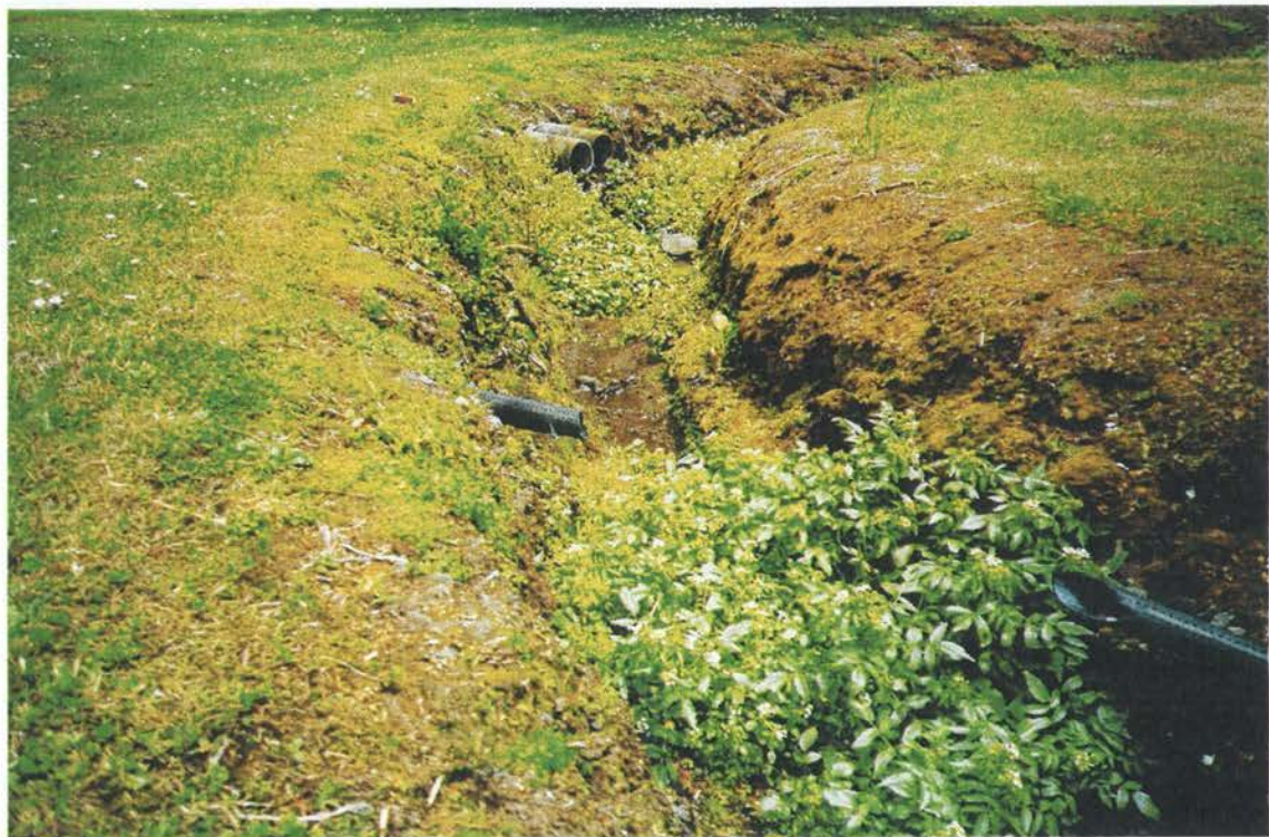
Plate 2: Site TN1 - Stormwater outlets to Tanners Point Reserve stormwater channel and in-channel vegetation.
