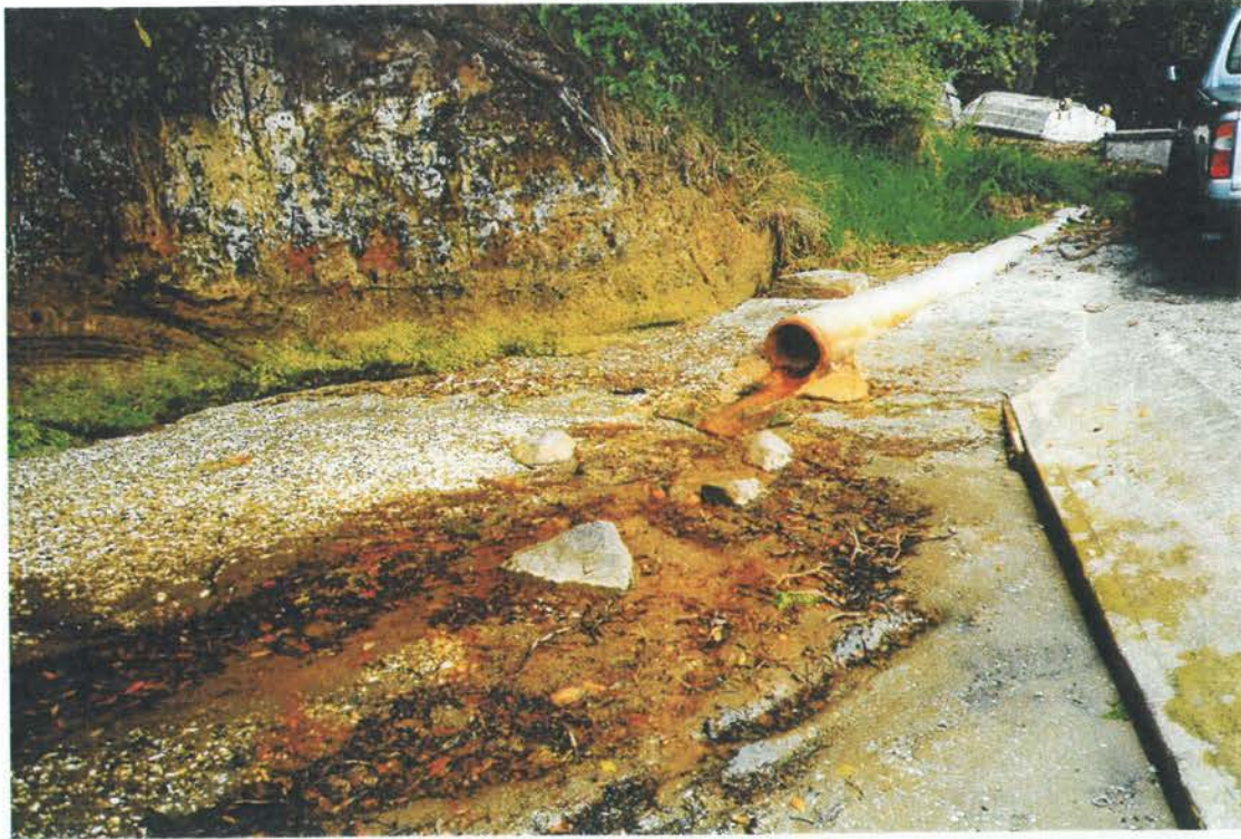
Plate 3: Site TN1 - Stormwater outlet at harbour margin from Tanners Point Reserve stormwater channel.
