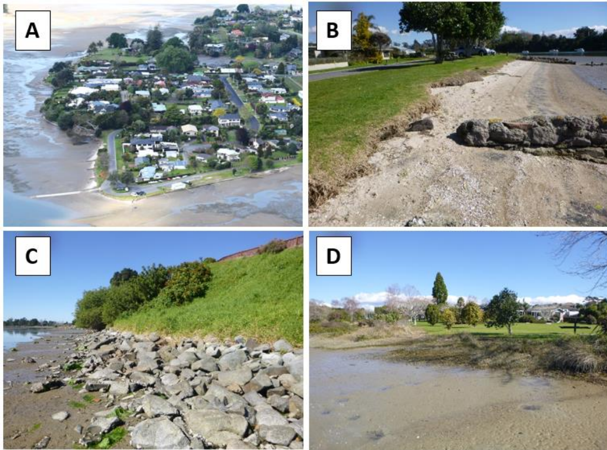
Figure 8-2 Site photos for Te Puna West. (A) Aerial shot of Te Puna West shoreline (Cells 8A & 8B), (B) groynes along the unconsolidated shoreline (Cell 8B), (C) revetment at the base of the cliffs (Cell 8C), (D) unconsolidated shoreline around Te Kopa O Te Hotu Reserve (Cell 8H).
