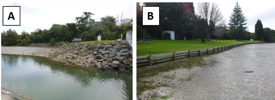
Figure 7-3 Protection structures at Plummer's Point. (A) Rock revetment, (B) timber seawall.
