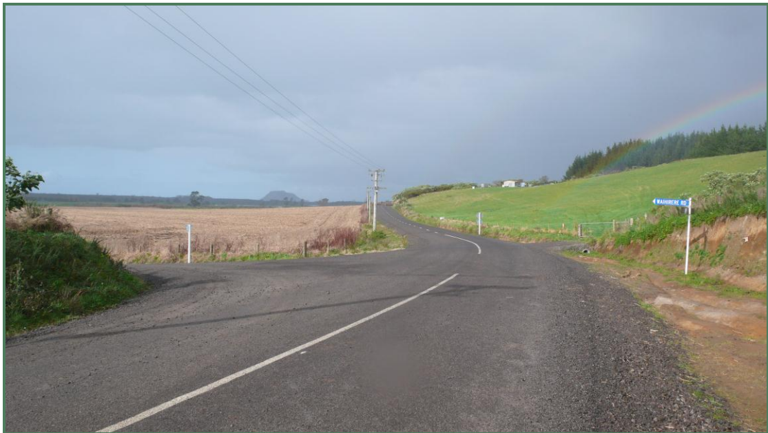
Photo 10: Matakana Road on core (sealed formation) looking South
