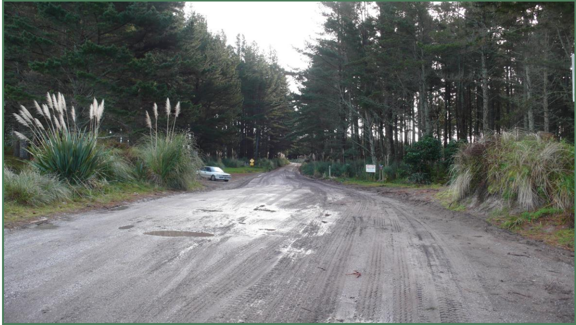
Photo 7: Right of Way formation looking North from Pane Pane Ramp
