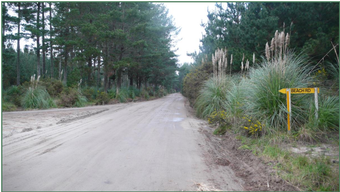
Photo 8: Main Right of Way (Hume Highway) unsealed formation on Barrier
