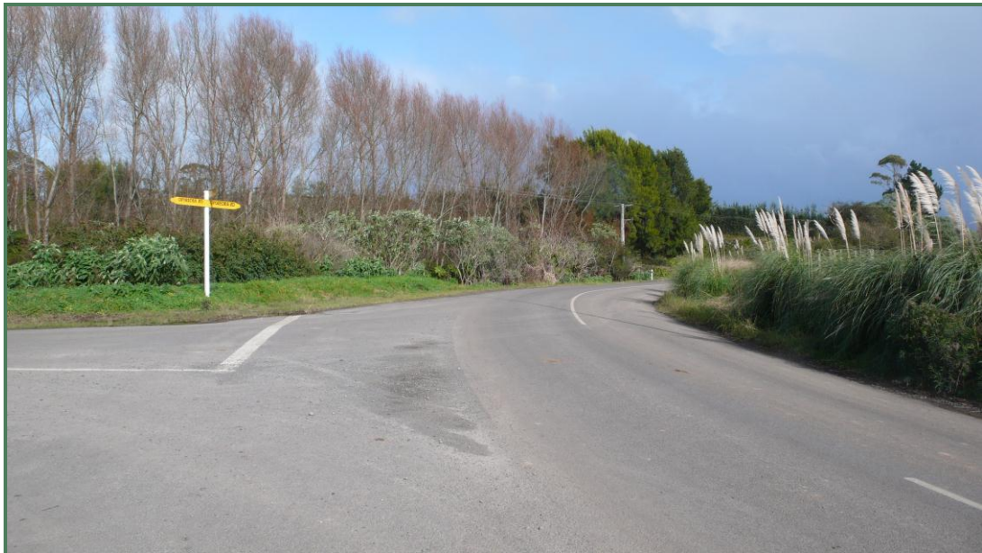
Photo 12: Oपुरeroa Road Intersection with Matakana Road (sealed formation)
