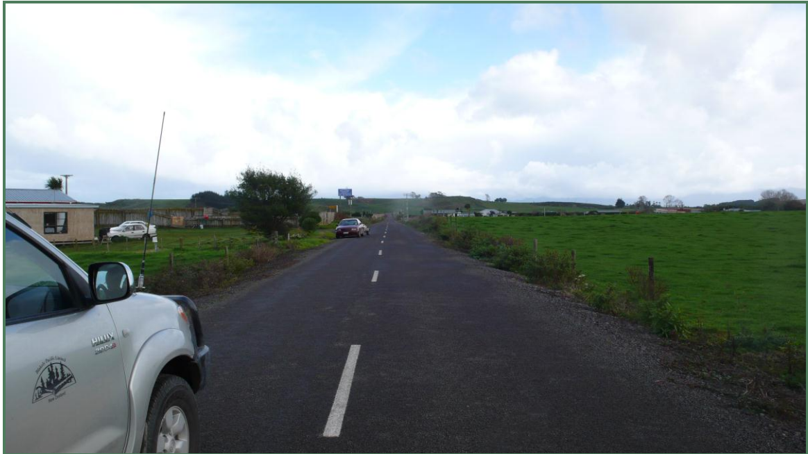
Photo 9: Waihirere Road sealed formation on Core
