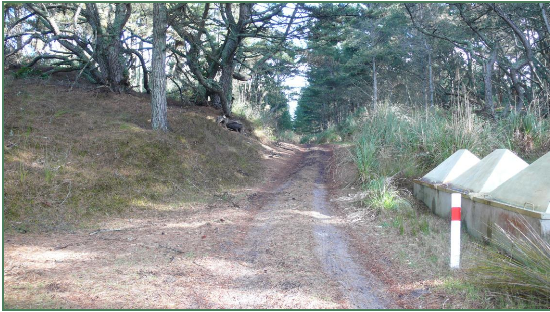
Photo 13: Pipeline Road (Right of Way) on Barrier (unsealed formation)
