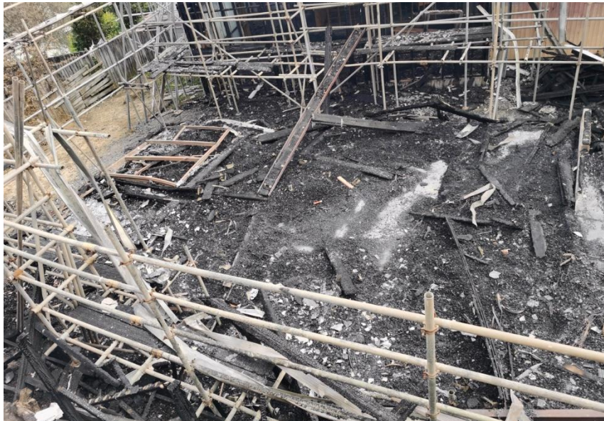
Figure 6: The extent of damage to Dwelling 3 – Overlook from South
