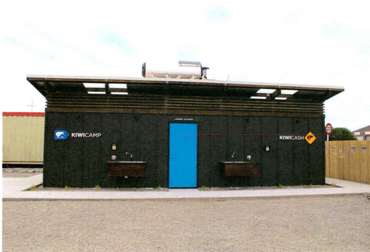
KiwiCamp® turnkey facility
