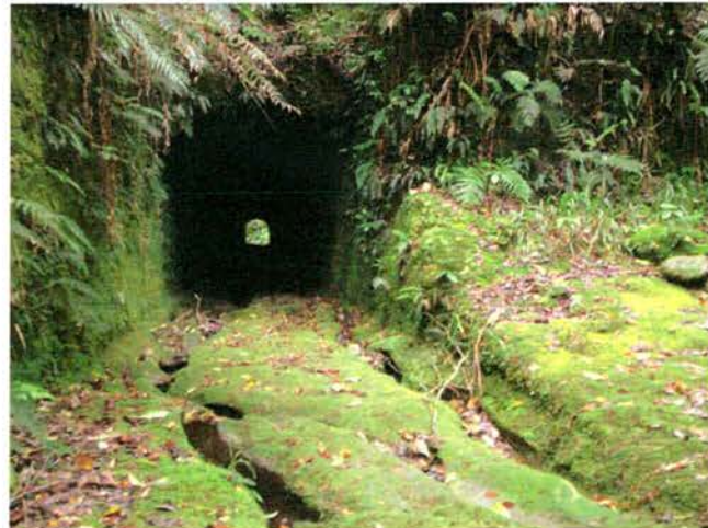
Caption: Te Rerenga Stream Tunnel under Pyes Pa Road (SH36)
