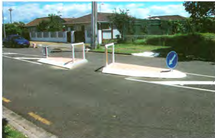
Typical pedestrian refuge layout. (Note. Highway lighting not included in photo)
