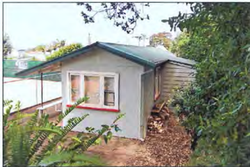
A new proposal to tidy up the building at the back of the tennis club. PHOTOS / MELANIE CAMOIN.
