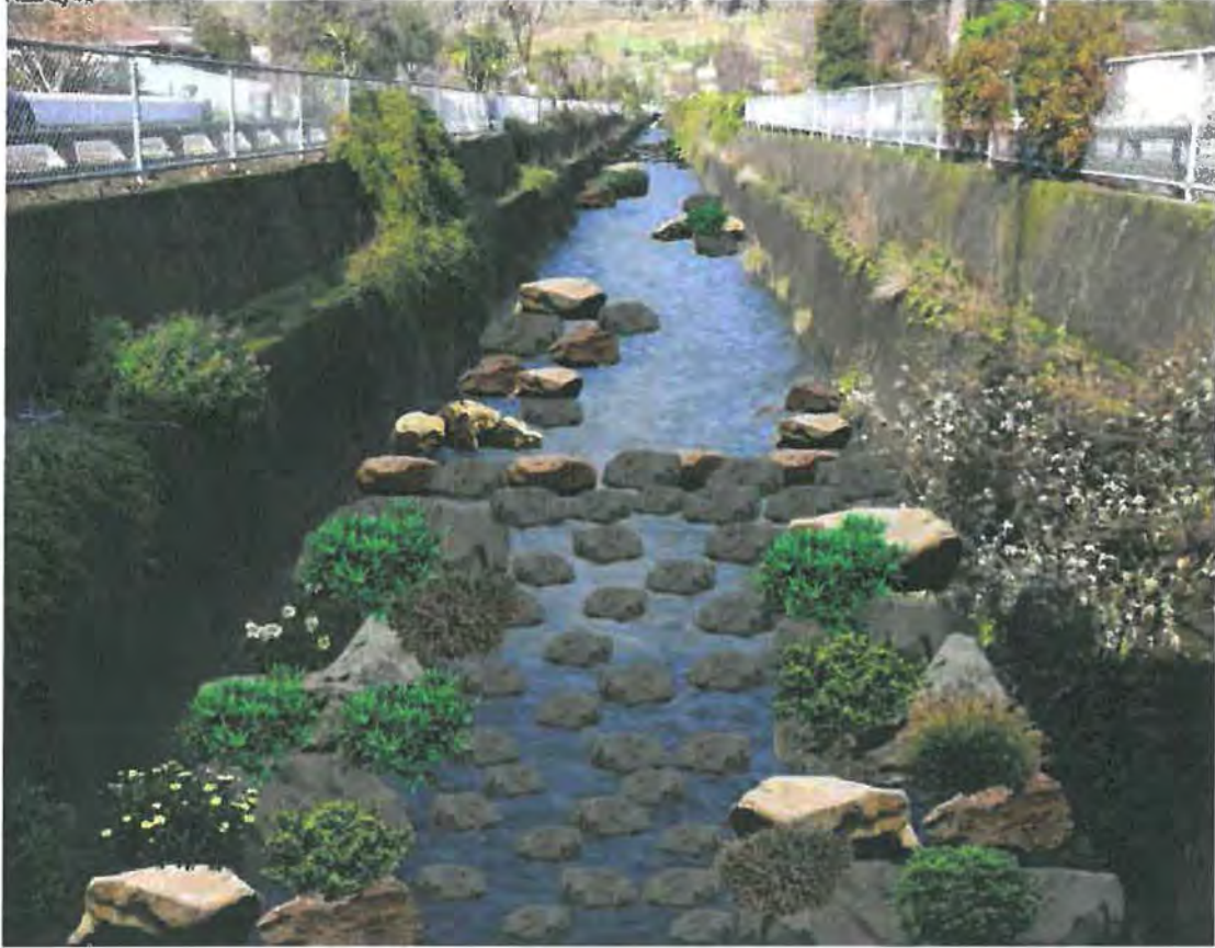
Visualisation of a constructed habitat sequence within a concrete lined channel. In this example a riffle – pool – run sequence with a meander using grouted rocks and deflectors is shown.
