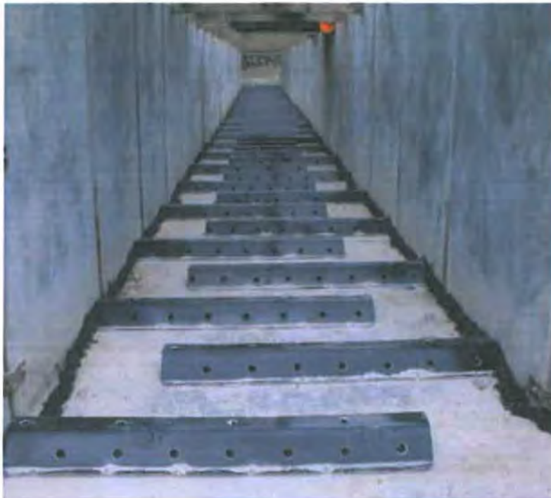
Fibreglass baffles example. Reference: http://fishladdersolutions.co.nz/fishway-baffles/
