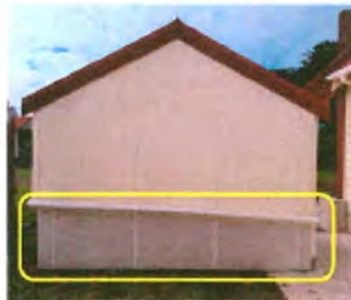
Whakaruruhaau: Repaired broken wall (yellow)
