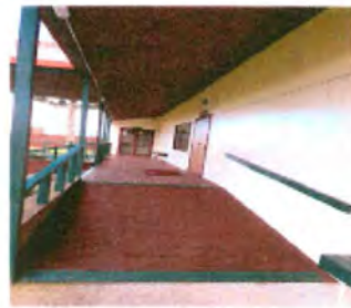
After: Front entrance into the Whare Kai.
