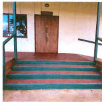
After: Front entrance into the Whare Kai.
