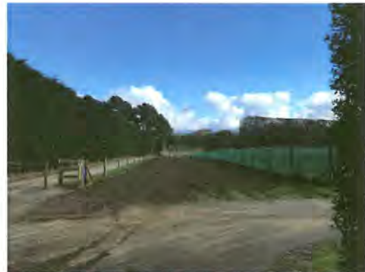
Carpark constructed at end of Newnham Road (11/07).
