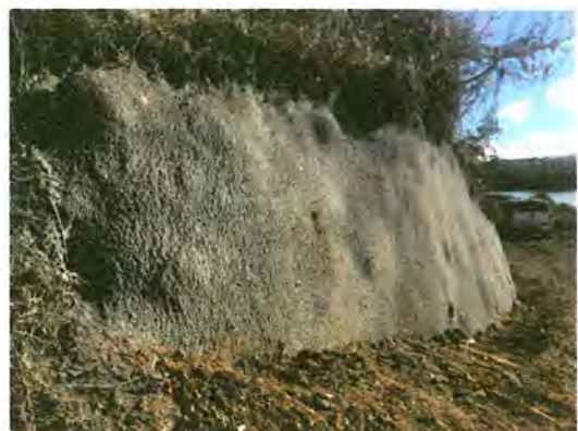
Construction of retaining wall adjacent Bridge 1 completed (11/07).
