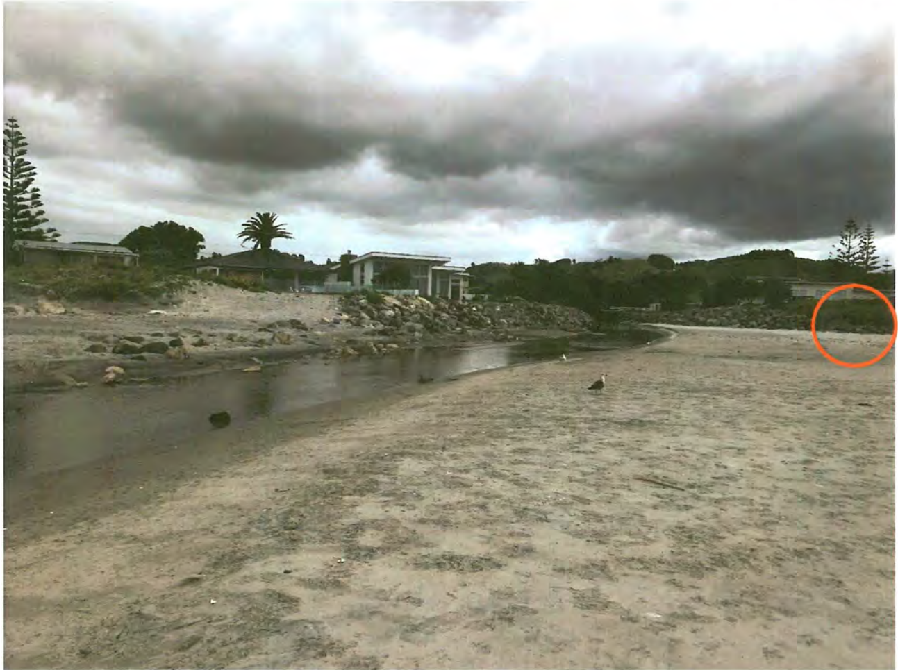
Figure 8 – Two mile creek showing rock training walls and northern seawall transition (red circle)
