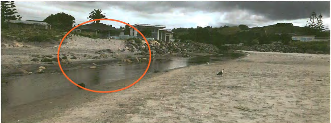
Figure 10 - Beach Access and Dune Tie-In (red circle)
