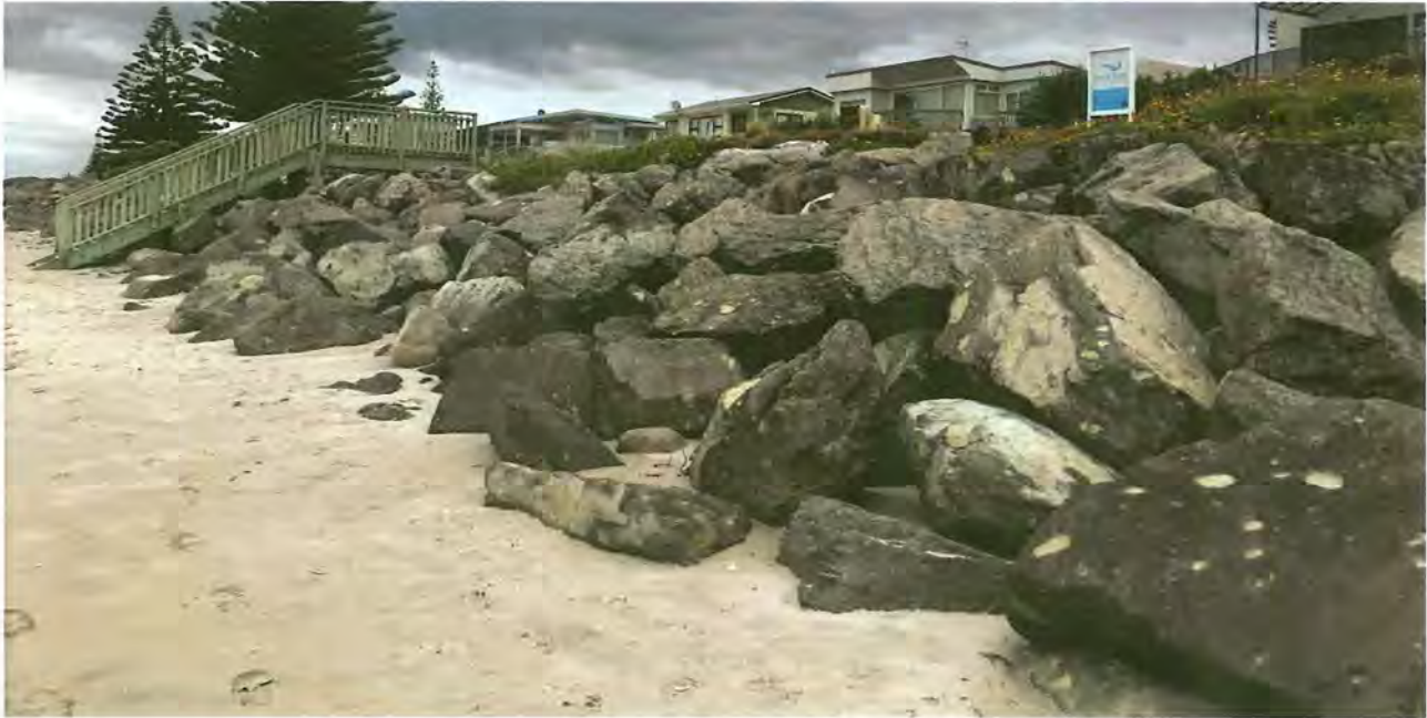
Figure 12 – Seawall Condition and Slope (Section C-C)
