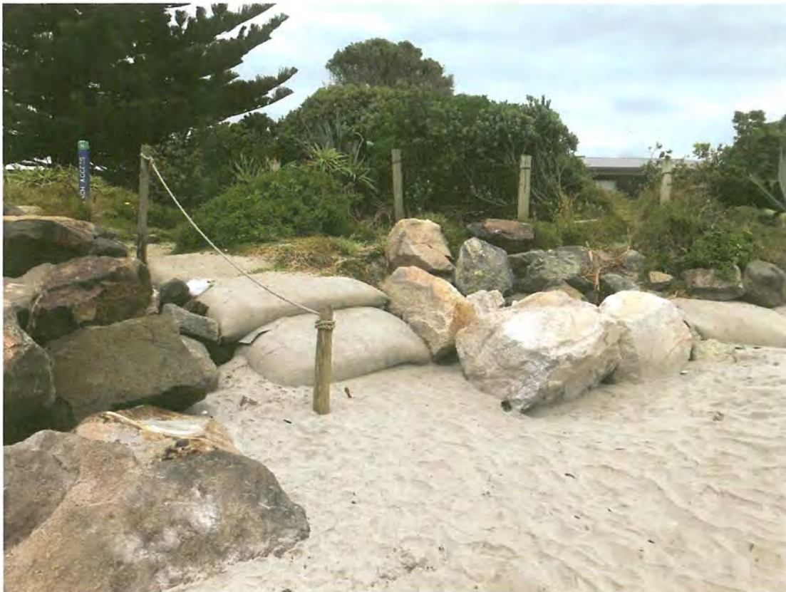
Figure 7 - Northern Seawall Northern Termination
