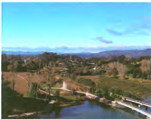
Plummers Point Scenic and Commuter Routes nearing completion (courtesy of Kotuku Landing video).
