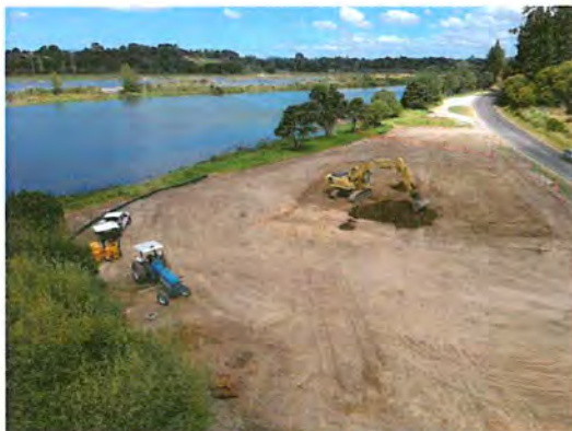
Construction of Pukewhaanake carpark underway 12 February 2019 (photo courtesy of WBOPDC website).
