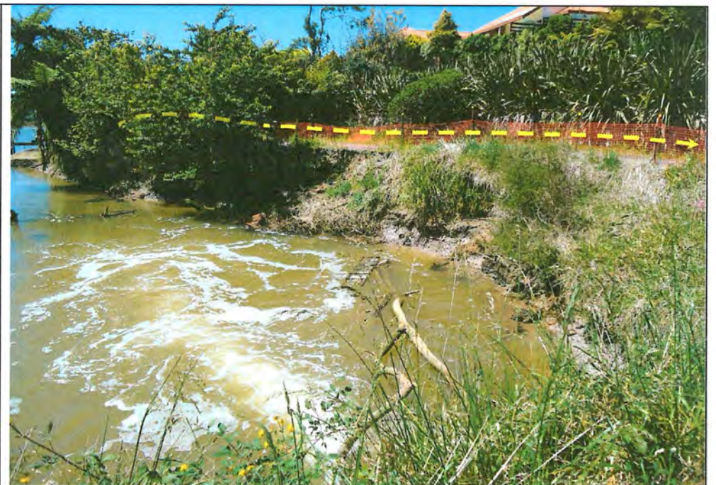
Photo 21: Passes alongside eroding embankment caused by culvert from the wetland inside the stopbank. The erosion, and culvert replacement by means of a flat-rack bridge & rock armouring, is currently being addressed with BOPRC and WBOPDC, via resource consent procedures.
