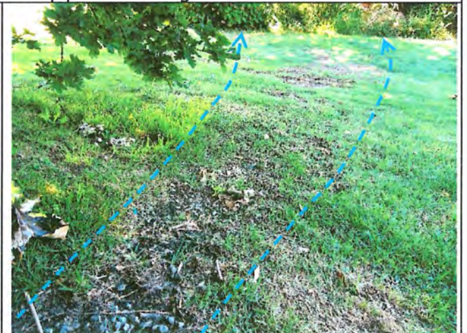
Photos 24 to 26: Stormwater outlet from neighbour at 56 Levley Lane discharges onto ground at landward edge of esplanade reserve with resultant outwash scour across walkway. This outlet needs to be extended to harbour-edge vegetation via a buried pipe at the neighbour's cost.
