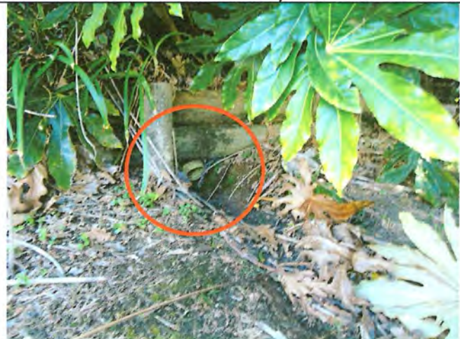
Photos 24 to 26: Stormwater outlet from neighbour at 56 Levley Lane discharges onto ground at landward edge of esplanade reserve with resultant outwash scour across walkway. This outlet needs to be extended to harbour-edge vegetation via a buried pipe at the neighbour's cost.
