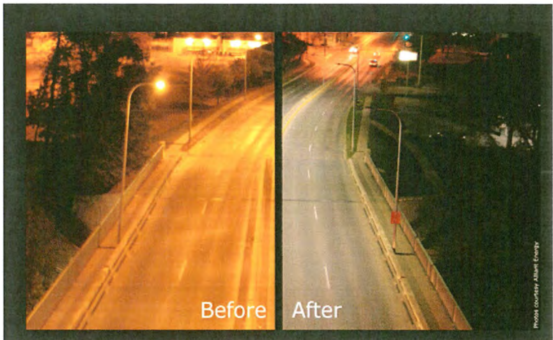
Picture 2 - High Pressure Sodium Luminaires and LED Luminaires
