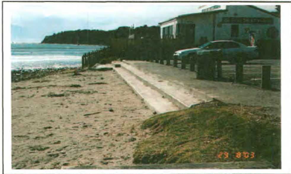
General View of Completed Gabion Protection Works
