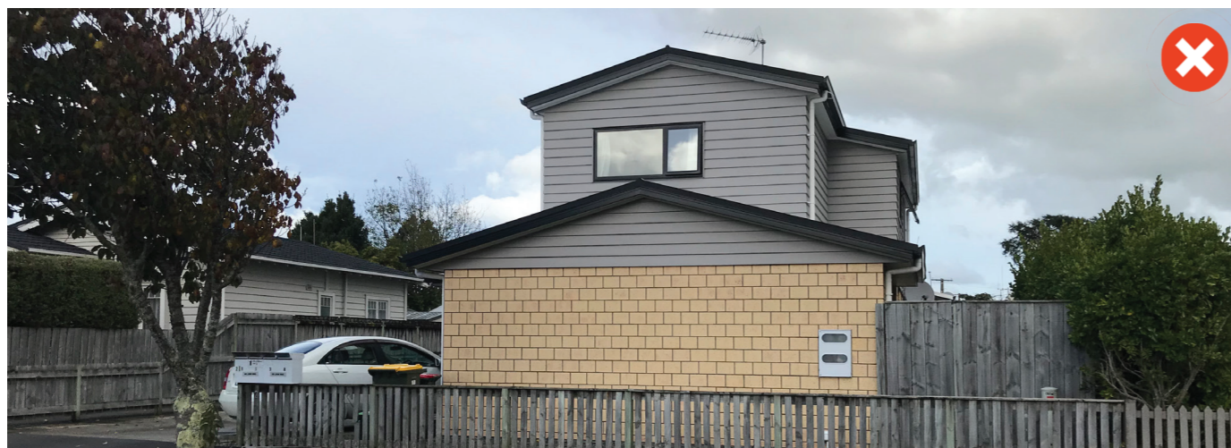
The windowless garage wall fronting onto the street results in no passive surveillance for pedestrians, a lack of legibility for visitors and if replicated along the street; a monotonous streetscape.
