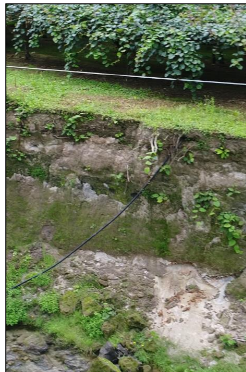
Image 1 - Example of erosion encroaching on Kiwifruit orchard at Ohineangaanga Stream.
