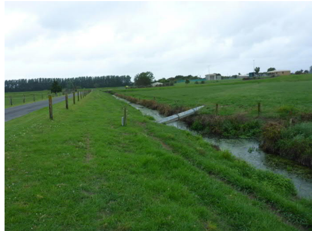
Stream 3 – Cannell Farm Drive waterway TP 3B (downstream)
