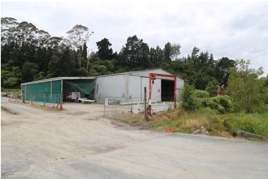
Plate 3: Light industrial land use situated between Te Puna Station Road and the ECMT.
