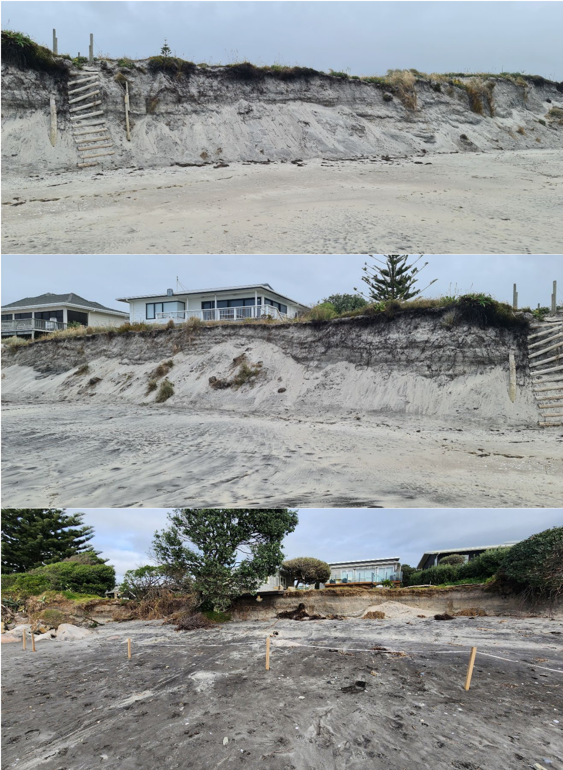
Figure 2: Examples of dune erosion issues at Waihi Beach (all above sites were later successfully managed using dune repair).
