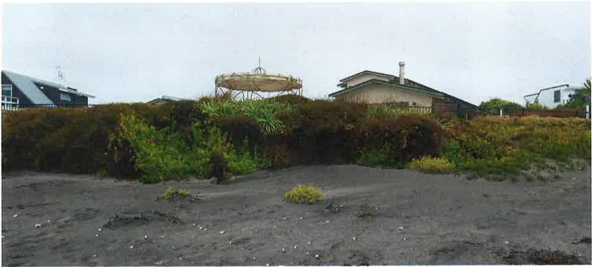
Photo 9: Shows remains of old seawall in front of 16 Glen Isla Place. 23 January 2025.
