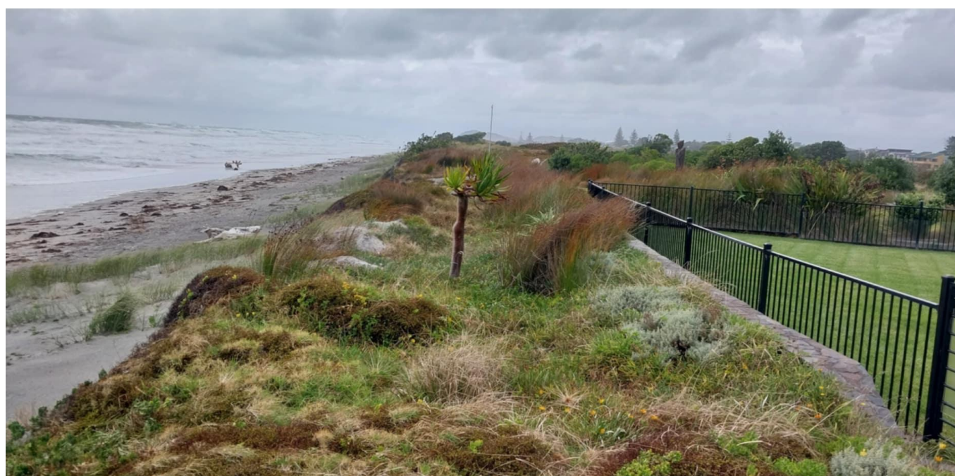
Figure 9 – Existing Dune 16, 14 and 12 Glen Isla Place Waihi Beach showing a great rate of natural dune repair – Feb 2025.
