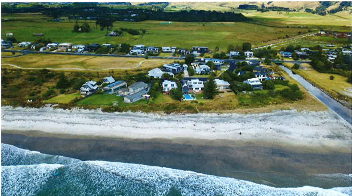
Photo 1: 23 January 2025, shows the current condition of the beachfront at Glen Isla Place.
