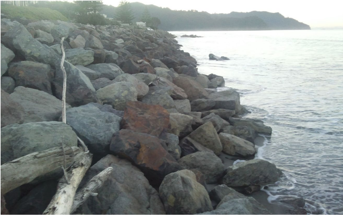
Figure 3: Seawall on Waihi Beach showing the absence of beach at high tide
