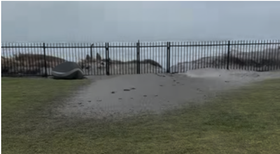
Image 5 (17 April 2025): showing sand blown over the dune onto the lawn of 12 Glen Isla Place.
