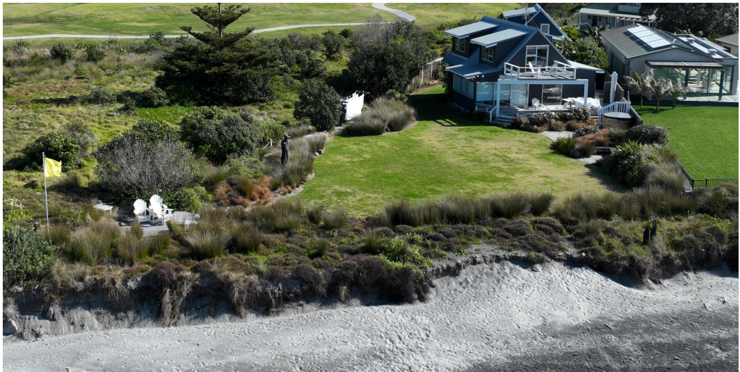
Image 3 (1 September 2023): after the storms of early 2023, the area of concern starting to erode more than the surrounding dune.
