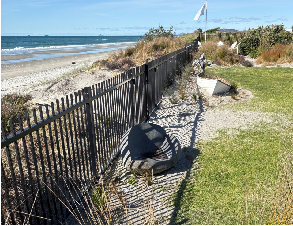
Image 10: shows the completed fence and replanting of the affected area inside the property.
