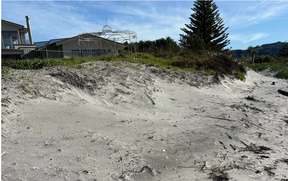
Image 8 (22 July 2025): plants that appear to have been sand covered and storm damaged in the dune seaward of 16 Glen Isla Place.
