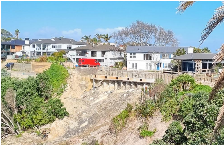
Photograph 1 Exposed Palisade wall
