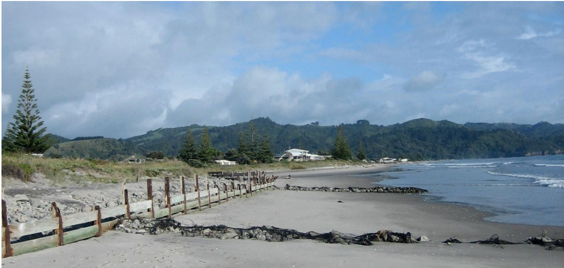
Figure 2: Remnant seawall prior to the 2010/2011 coastal protection works.
