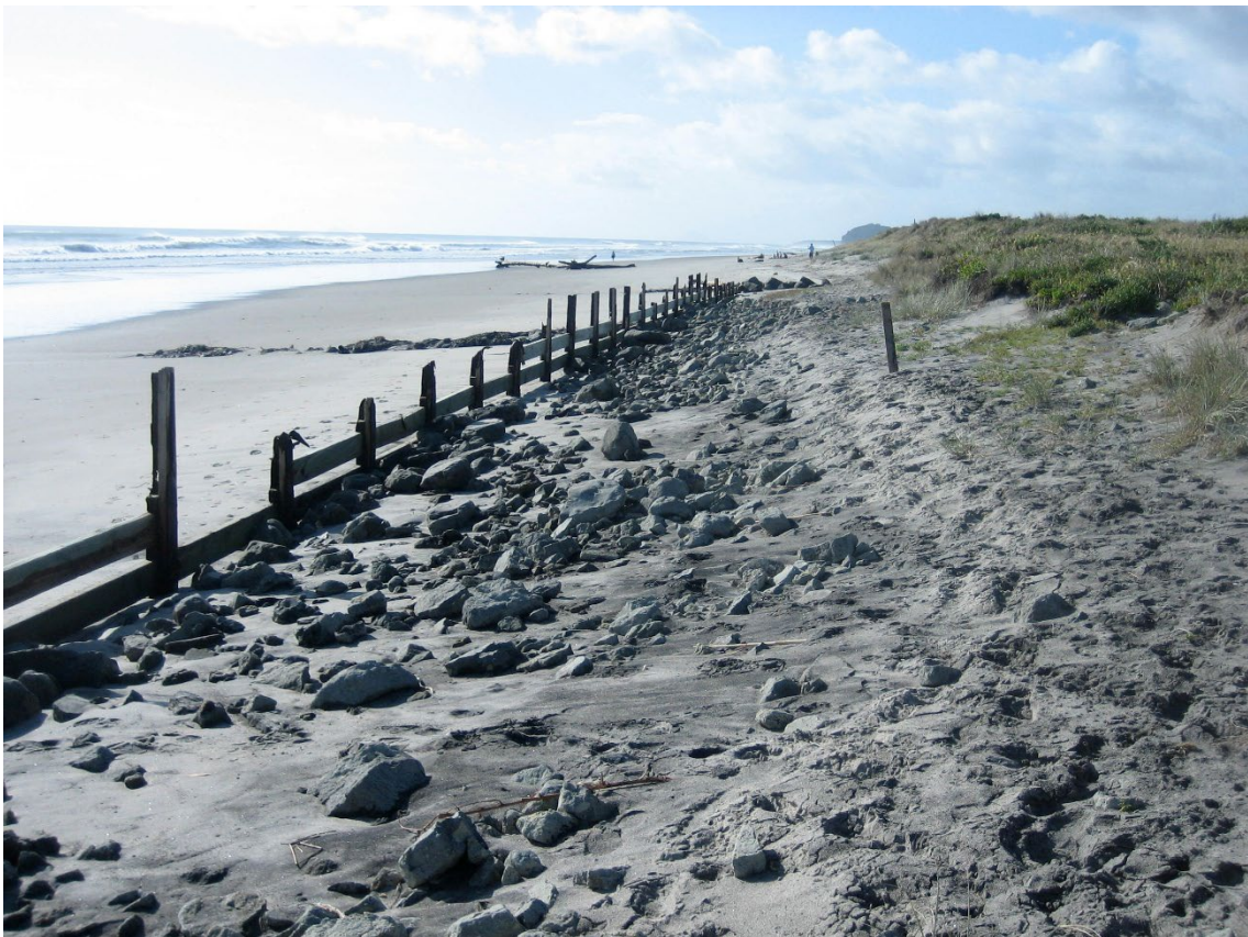
Figure 1: Remnant seawall prior to the 2010/2011 coastal protection works.
