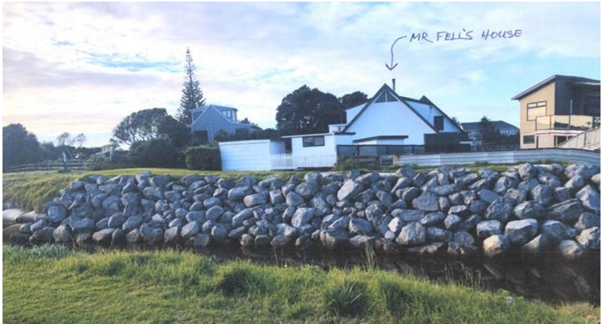
Image 1: Seawall constructed by Beach Contractors in 2023 in Three Mile Creek in front of 7 Glen Isla Place.
