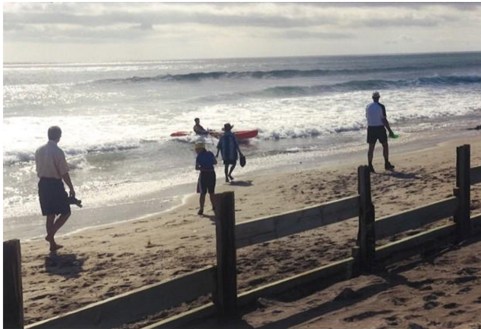
Image 1: The Glen Isla seawall built in 1983 (date of photo unknown but between 1997 and 2011)
