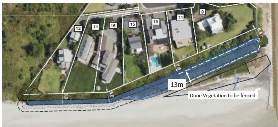
Figure 5.0a: Indicative area of vegetation requiring removal
