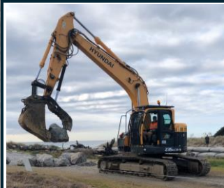
CATERPILLAR TRACKED EXCAVATORS MOVING ALONG CREEK PLACING ROCKS TO WALL
