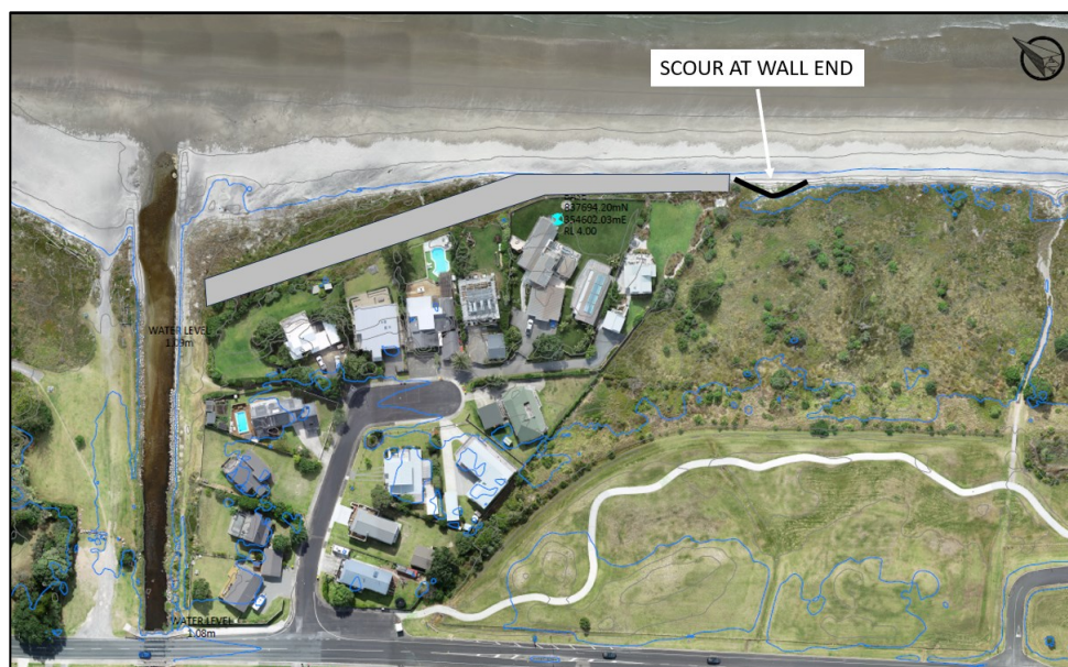
Figure 23: Potential scour at southern wall end
