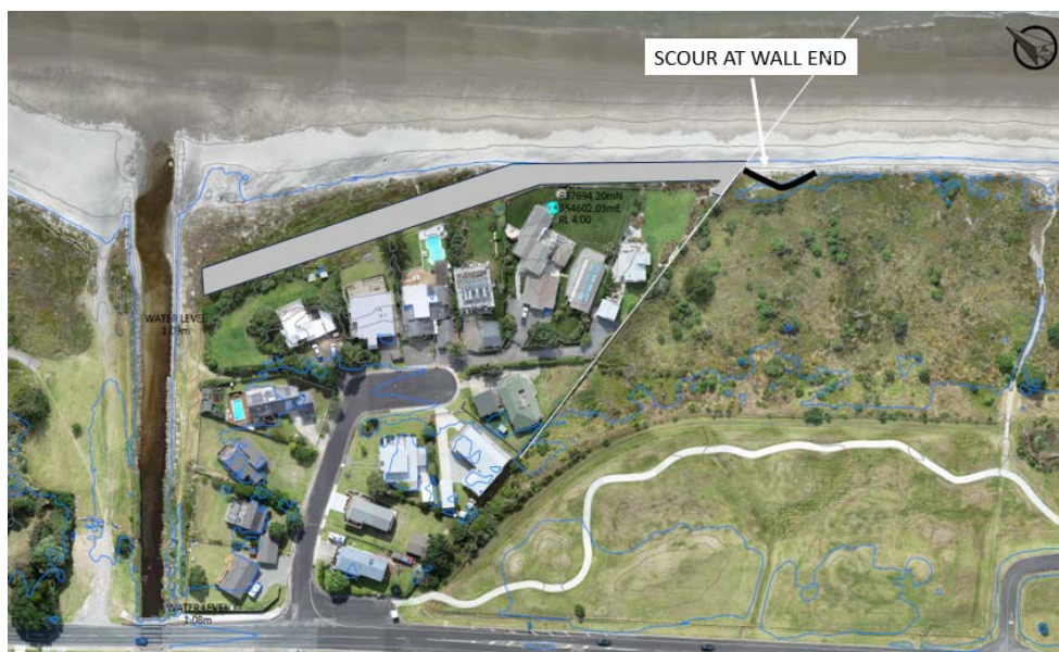
Figure 5.3.2c: Potential scour at southern wall end
