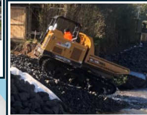
SMALL CATERPILLAR TRACKED MAROOKA CRAWLER WILL LIFT AND CARRY ROCKS TO EXCAVATOR
