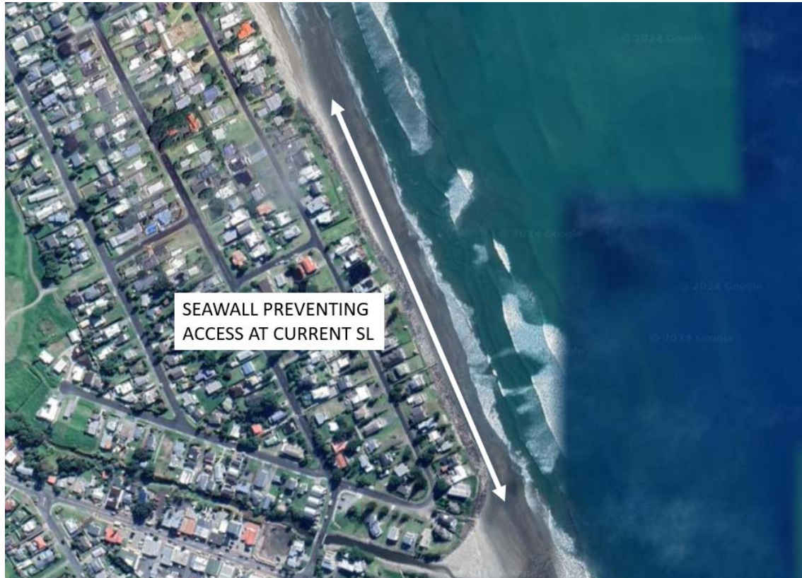
Figure 5.3.4b: Seawall at Shaw Road – water at wall
