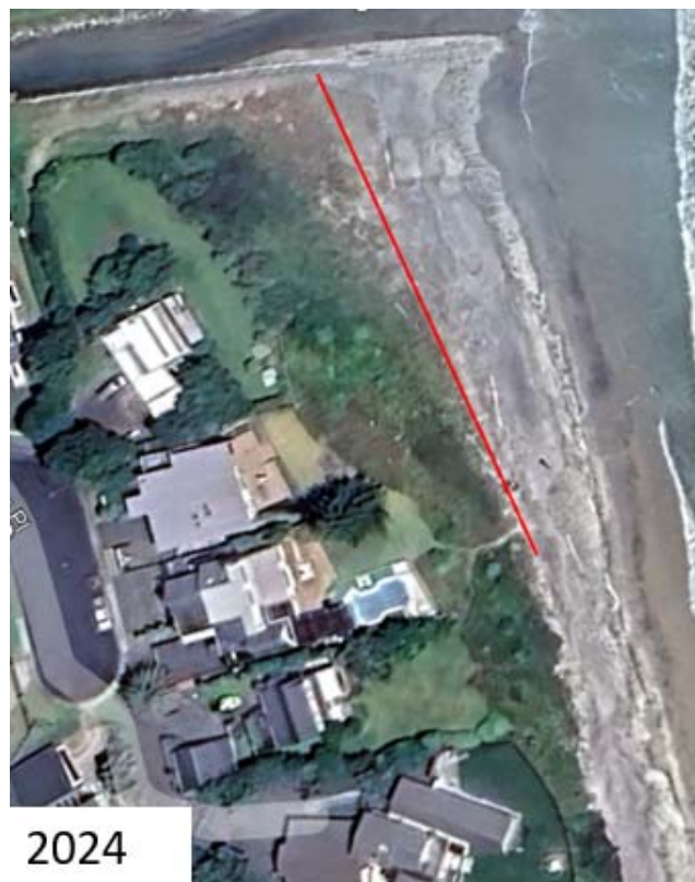
Figure 3.4c: Dune line post groyne construction
