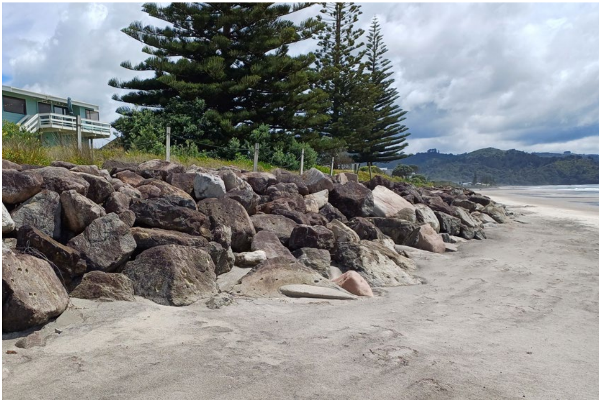
Figure 2: Example of a fully exposed seawall approximately 200 metres north of the site
