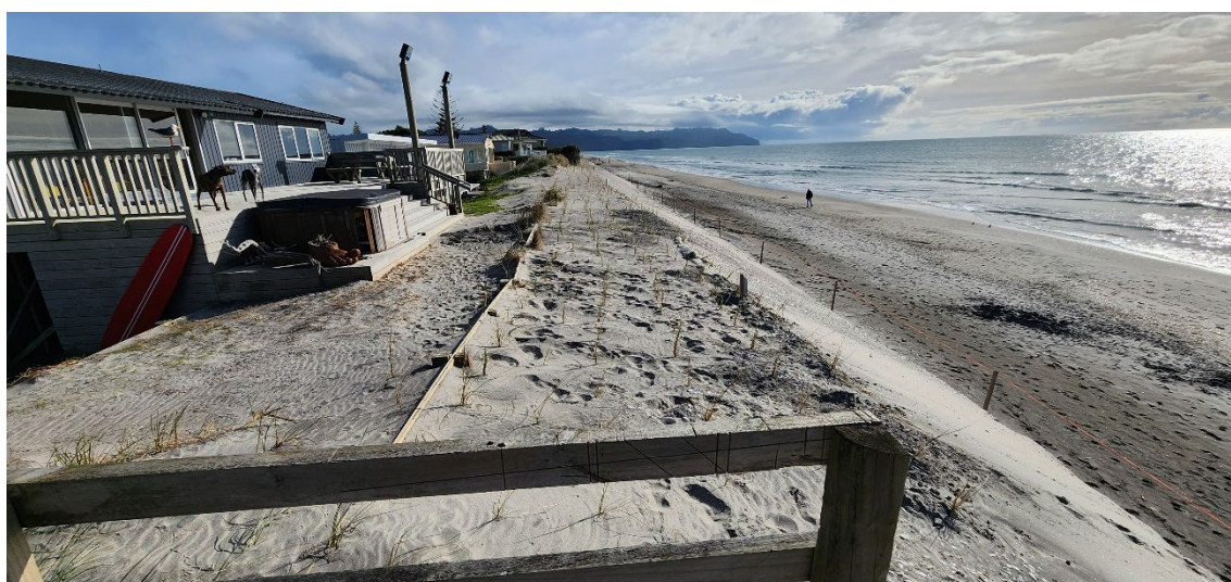
Figure 5: Example of dune repair using push-up - Broadway Road, Waihi Beach
