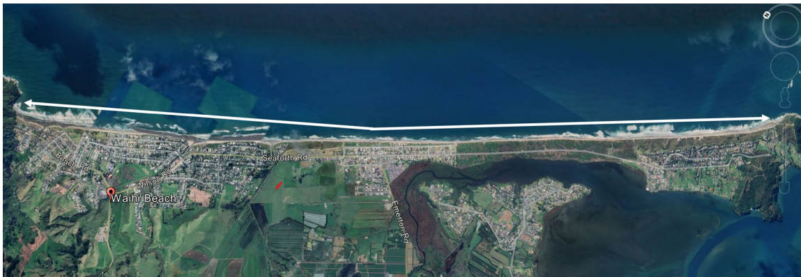
Figure 1: Area for which the consent for dune repair is sought.
