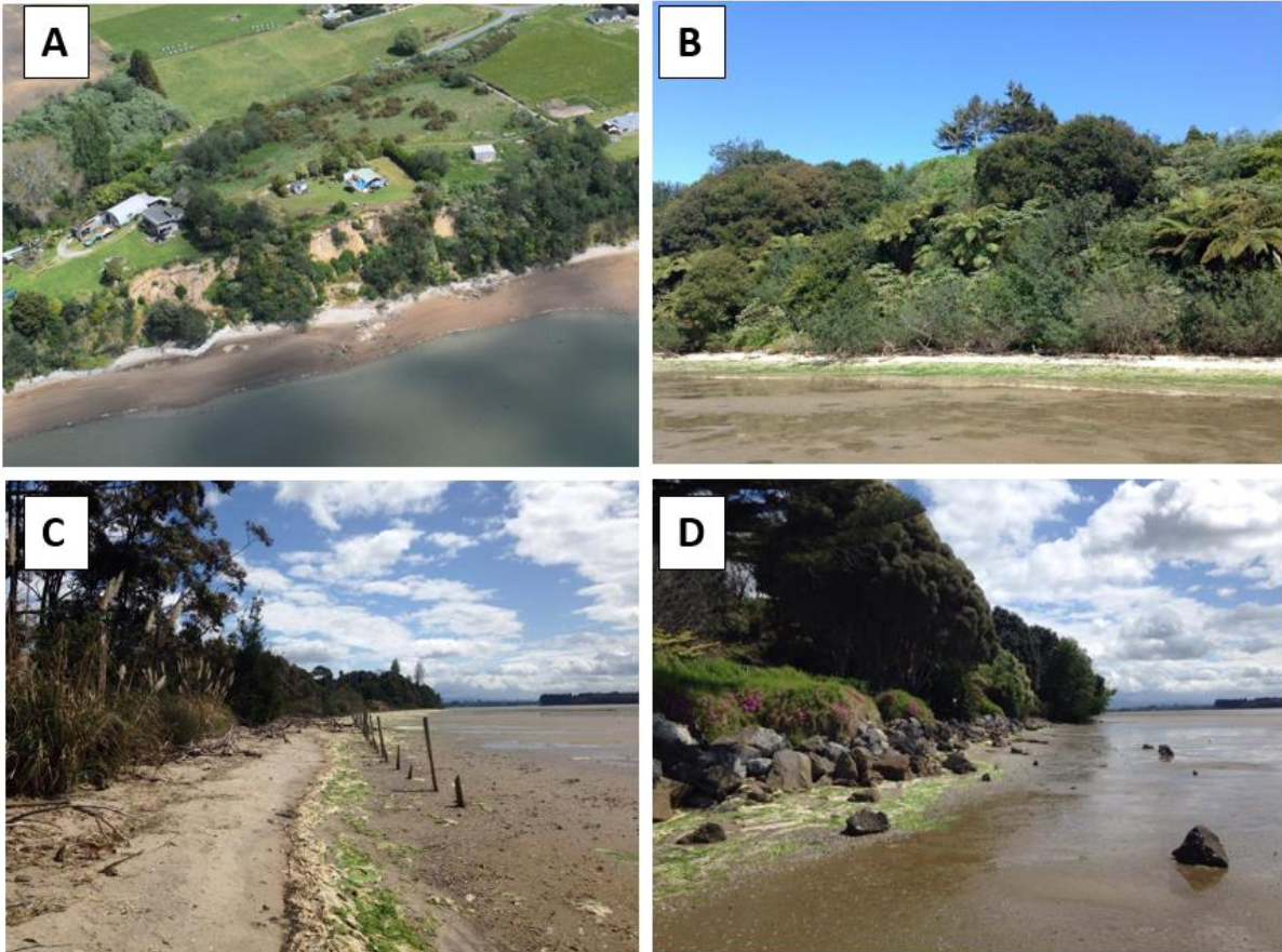
Figure 9-2 Site photos for Te Puna. (A) Exposed cliffs (Cell 9B), (B) stable cliffs with high tide beach (Cell 9C), (C) unconsolidated shoreline (Cell 9D), (D) low cliffs with rip rap (Cell 9F).
