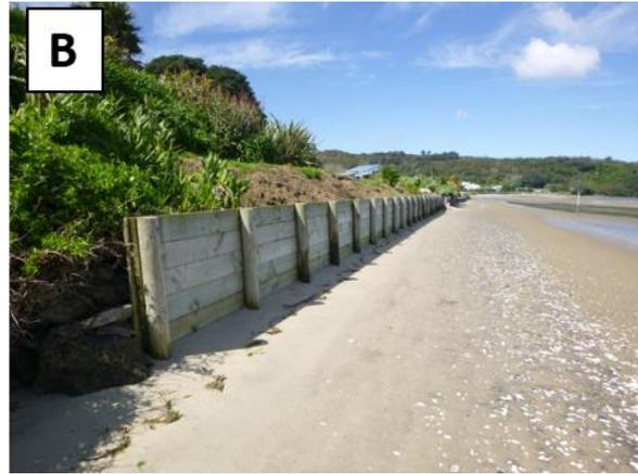
Figure 1-3 Examples of protection structures around the Bowentown shoreline. (A) Revetment along the grass bank (Cell 1C), (B) timber seawall (Cell 1D).
