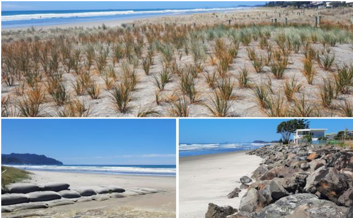
Figure 1.13: Example of protection structures and dune planting along Waihi Beach. (Top) dune planting in cell 1A. (Bottom left) Groynes at Three Mile Creek outlet. (Bottom right) rock revetment in cell 1D
