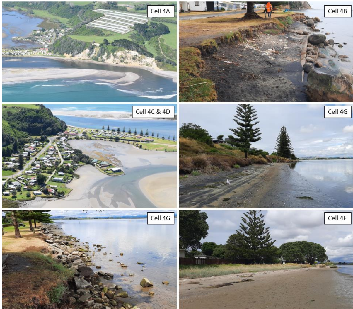
Figure 4.2: Site photos along the Waihi Estuary shoreline
