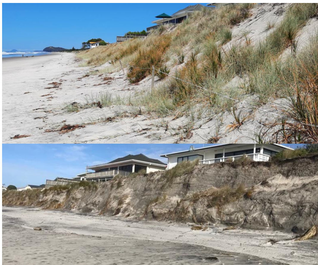
Figure 1.4: Site photos taken near profile CCS49, Cell 1H. (Top) 12 th February 2021 prior to the 2021 storm events (source T+T). (Bottom) 27 th May 2021 following the first storm event (source BOPRC)
