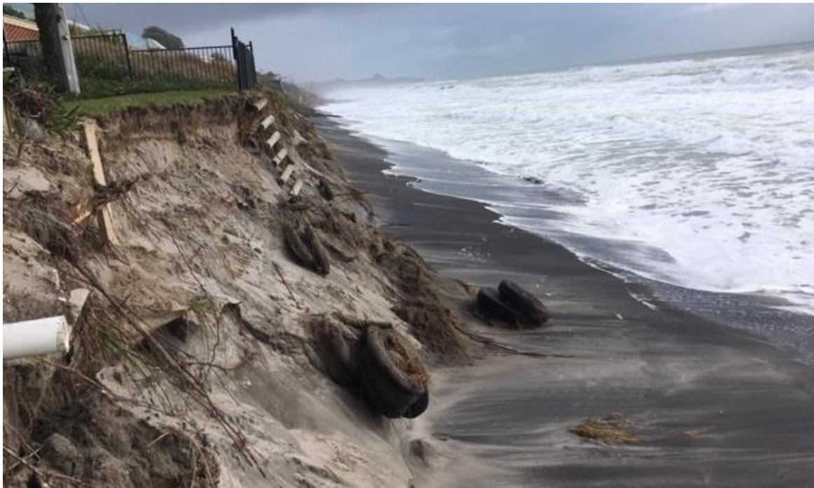
Figure 5.4: Example of recent storm erosion (21 August 2020) along Pukehina Beach near CCS27 (Cell 5D). Photo sourced from westernbay.govt.nz
