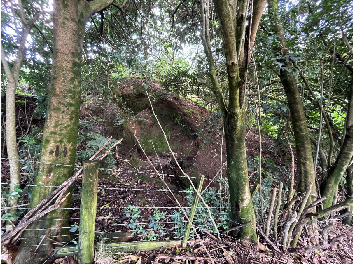
Figure 6 – View of Earthworks in Northwest Corner of Application Site
