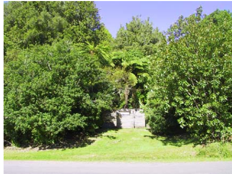
Toilet Block at edge of Puketoki Reserve
