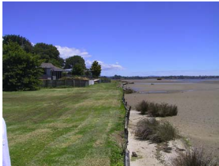
Existing seawall in reserve
