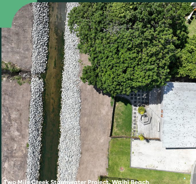
Two Mile Creek Stormwater Project, Waihi Beach
