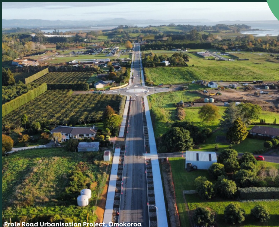
Prole Road Urbanisation Project, Ōmokoroa
