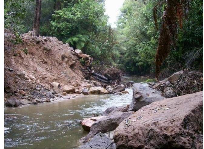
Road works 7km upstream of Oropi intake
