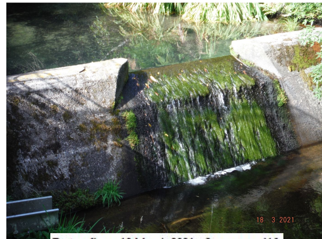
Tautau flows 18 March 2021 - 2 pumps - 416 l-s - Scour closed
