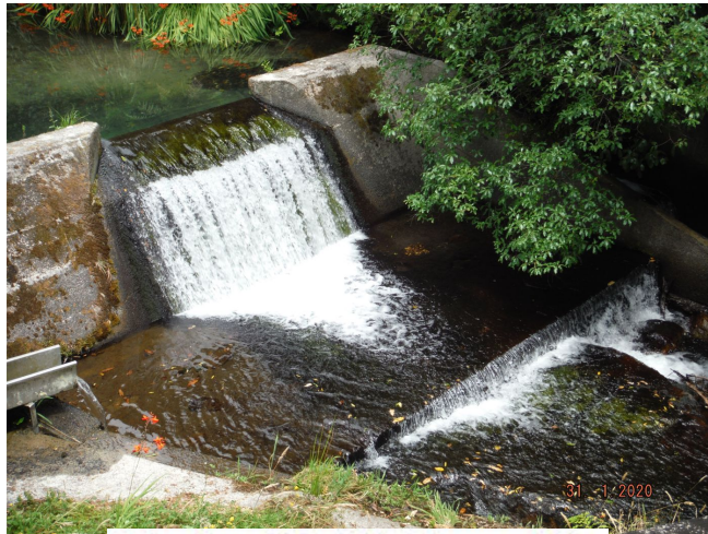
Tautau flows 31 Jan 2020 - 2 pumps 403 l-s scour closed
