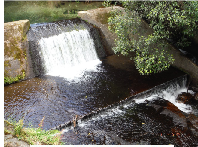
Tautau flows 17 Sep 2020 - 2 pumps - 416 l-s - Scour closed
